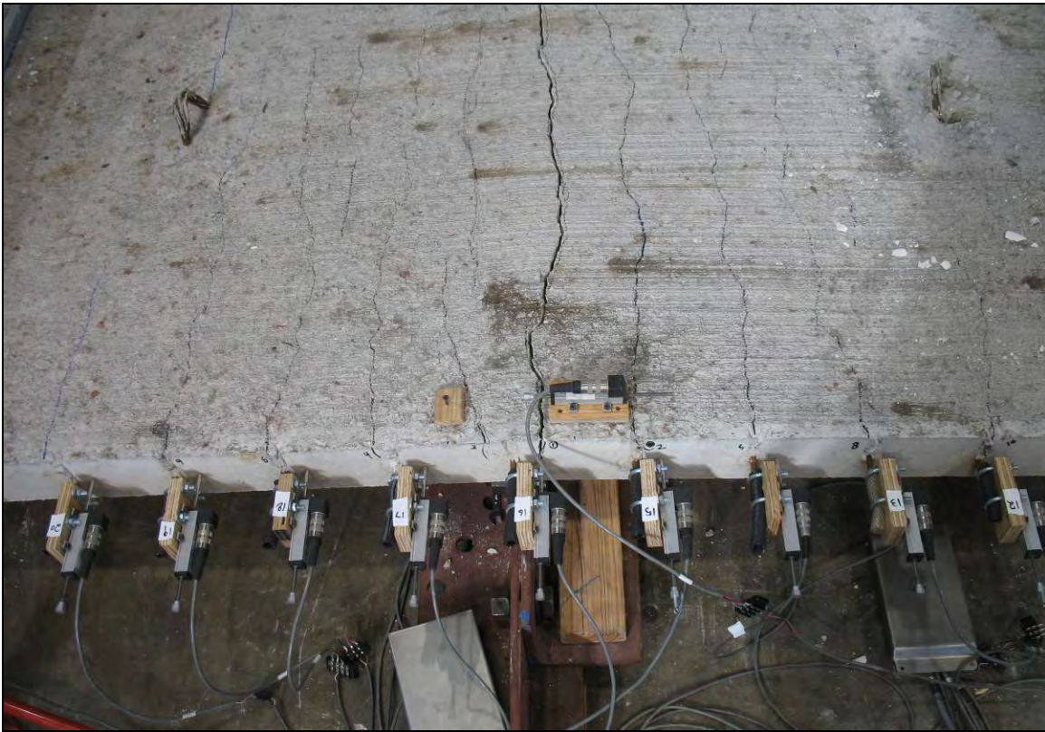
Figure 7.20 Edge of Specimen C3 after testing
