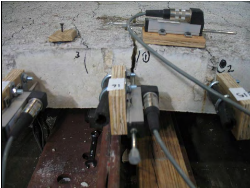
Figure 5.16 Gage 26 shown with the plunger stuck in the major crack of Specimen C3
