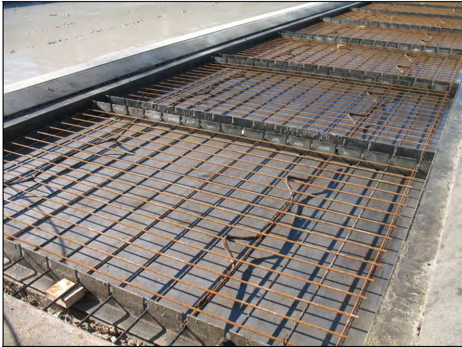
Figure 4.1 Transverse reinforcement in place at Plant A
