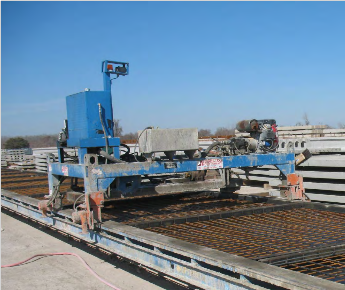
Figure 6.8 Vibrating screed used at Plant B
