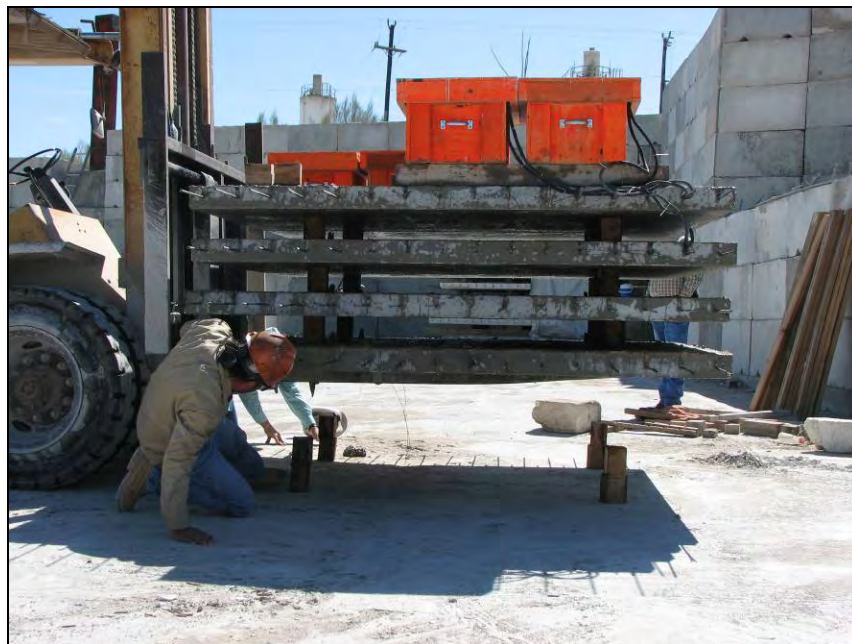
Figure 4.15 Stack of panels placed in storage area at Plant A
