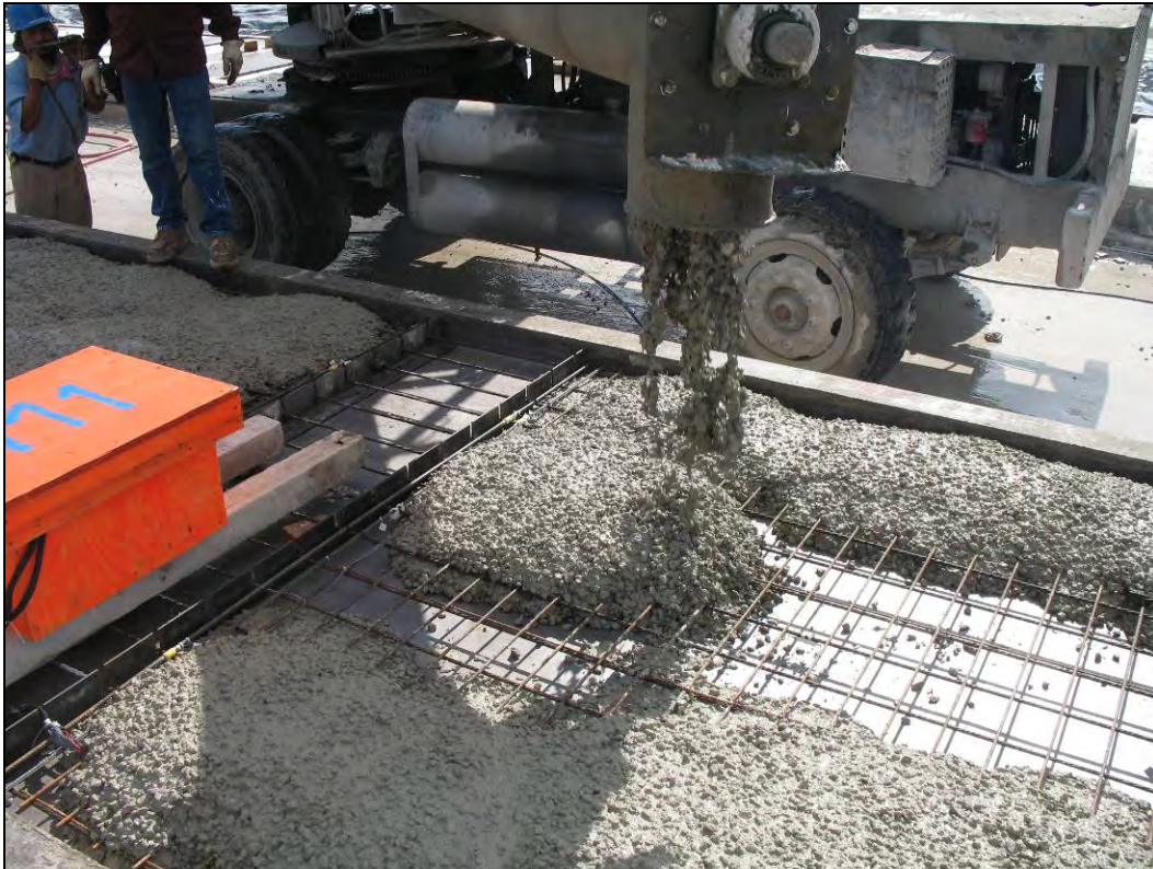
Figure 4.11 Sidewinder pouring concrete into forms and over gages at Plant A
