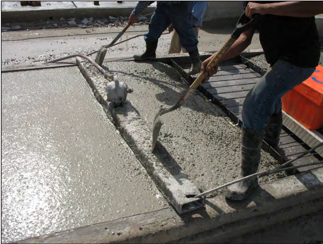
Figure 4.12 Plant A's crew running a vibrating screed over the wet concrete
