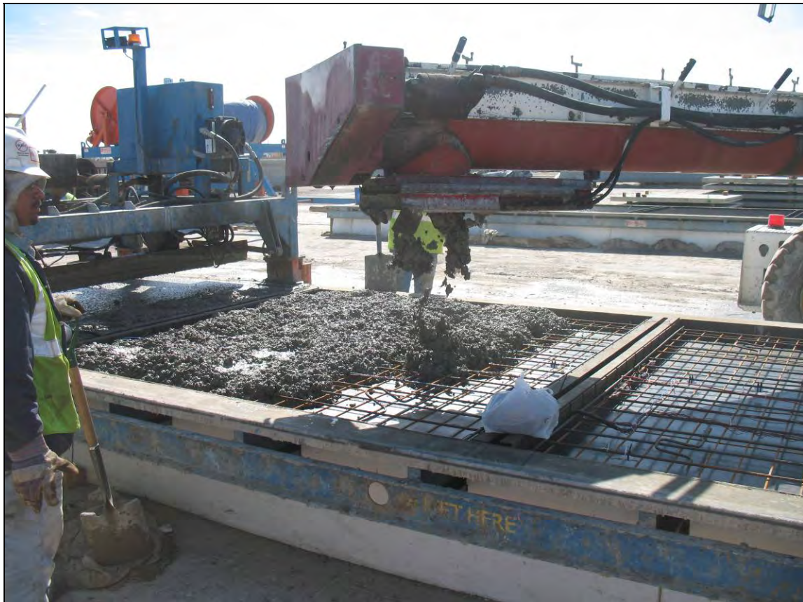
Figure 6.9 Sidewinder pouring concrete into forms and over gages
