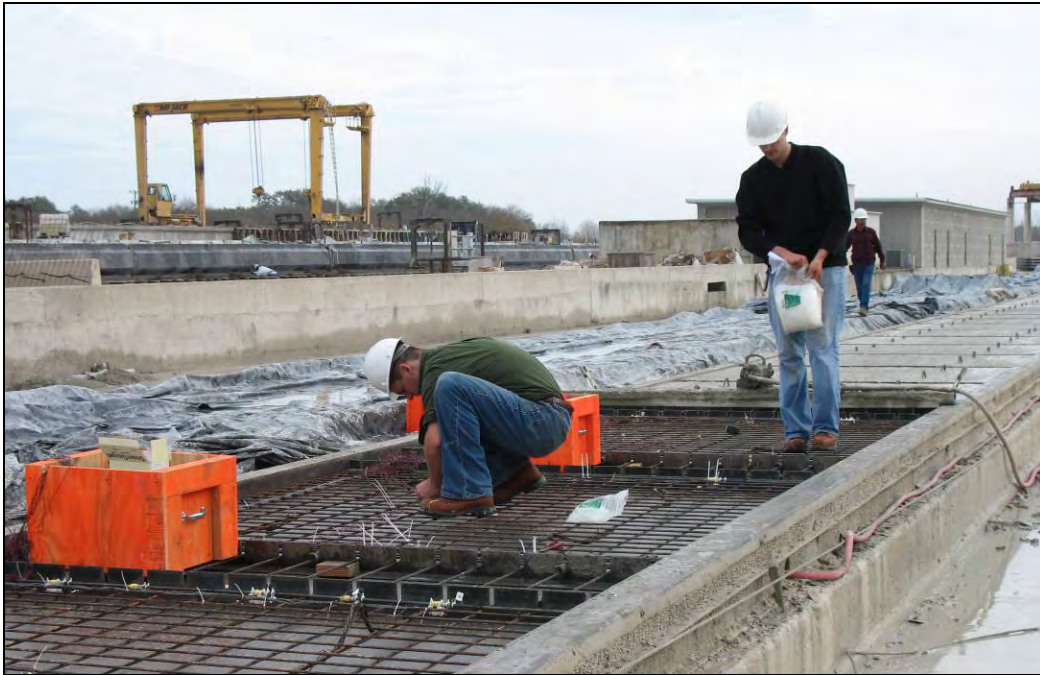
Figure 4.10 Installing gages at Plant A
