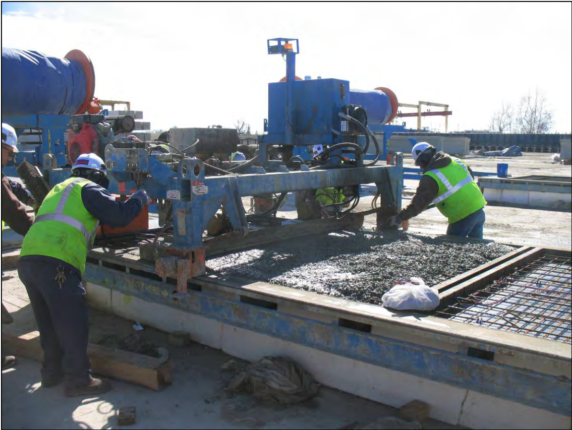
Figure 6.10 Vibrating screed being maneuvered over a panel at Plant B
