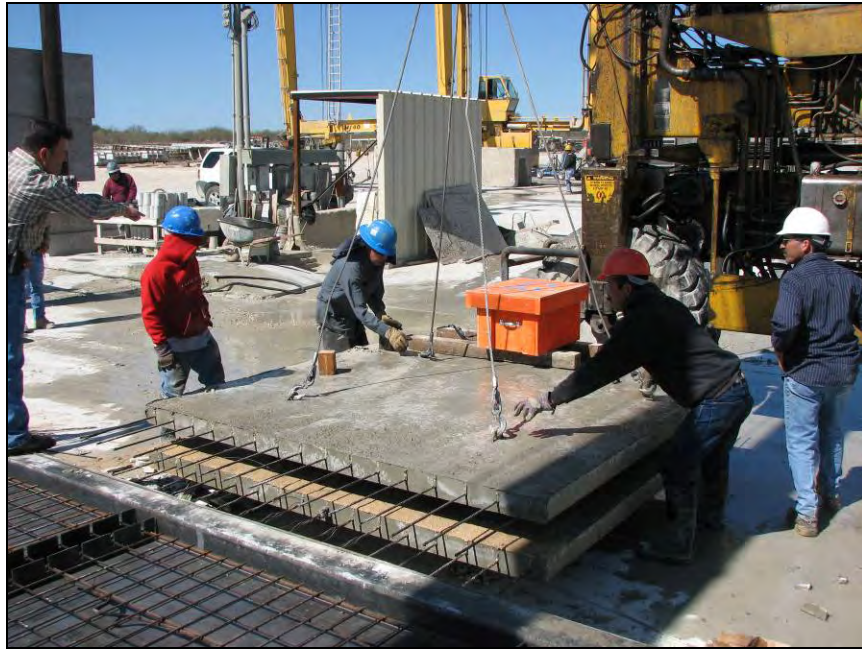
Figure 4.14 Panels lifted out of prestressing bed and stacked at Plant A
