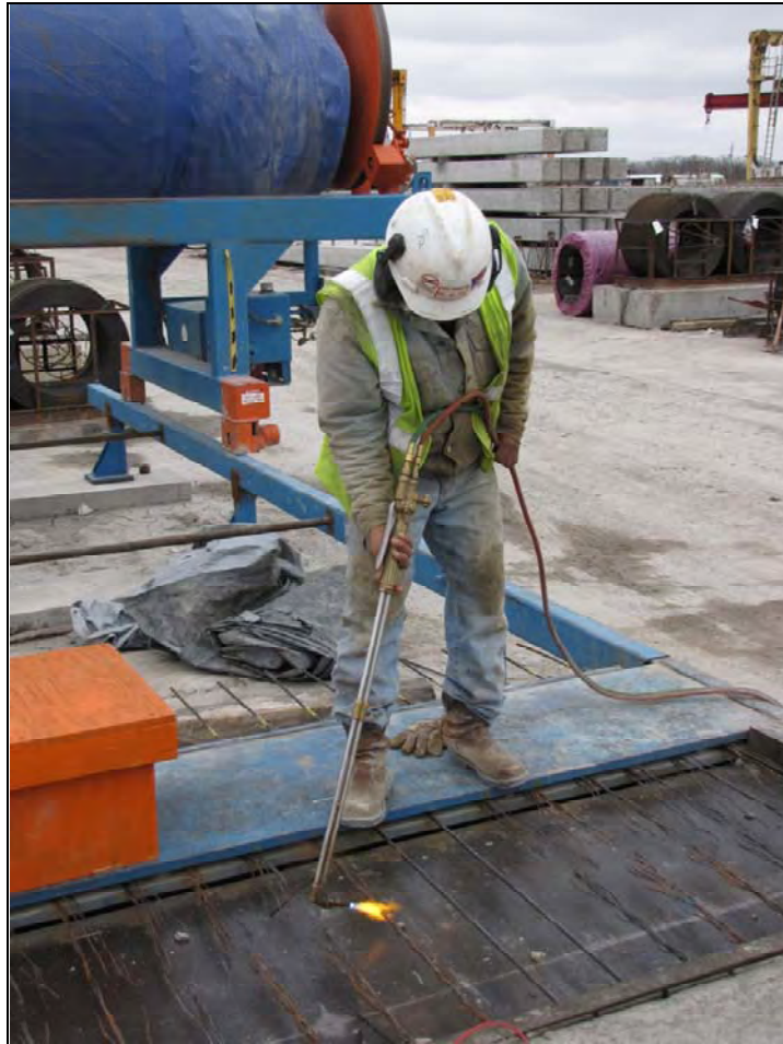
Figure 6.11 Strands being torch released at Plant B
