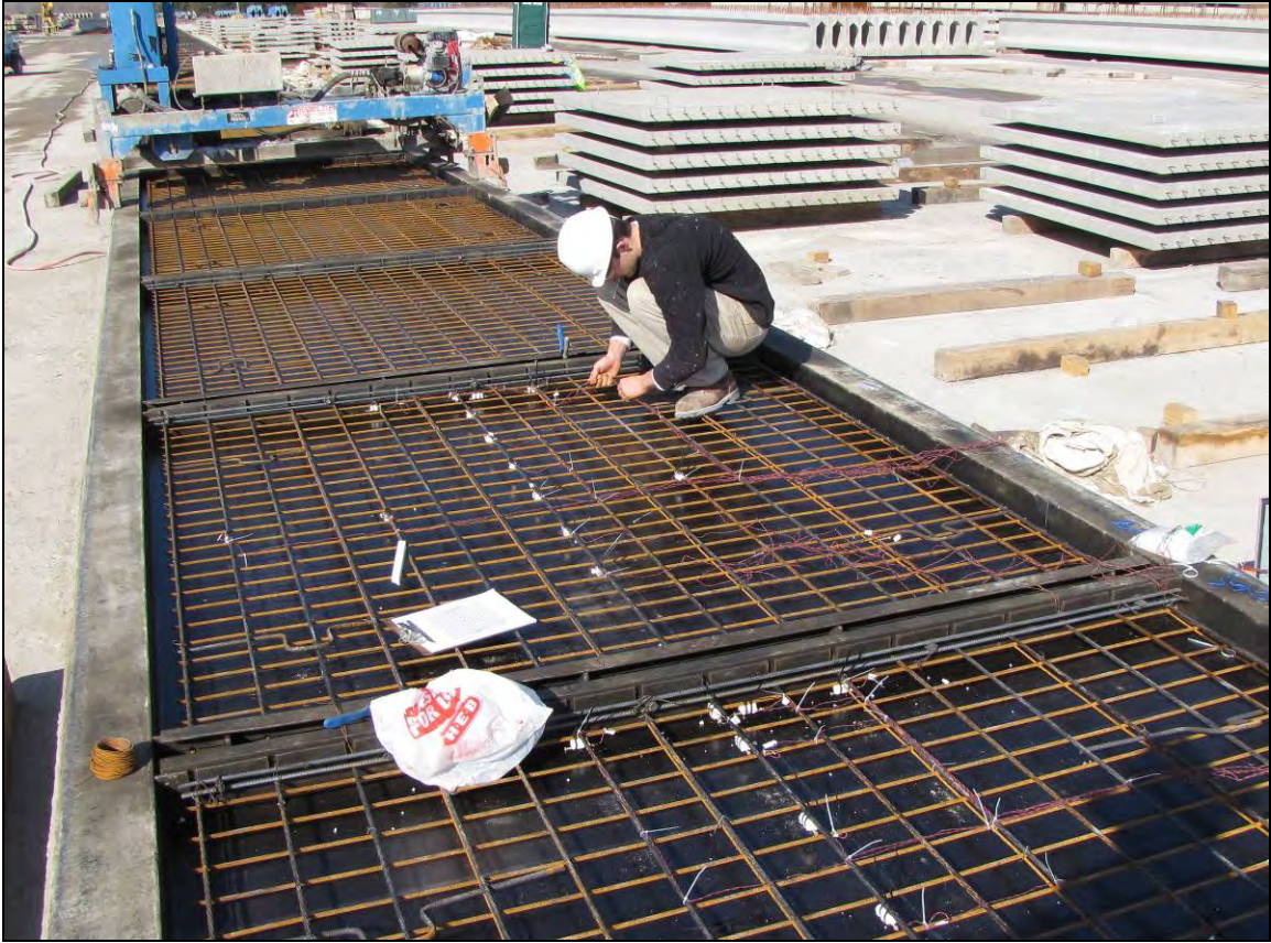
Figure 6.7 Installing gages at Plant B
