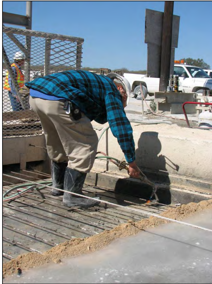
Figure 4.13 Strands being torch-released at Plant A
