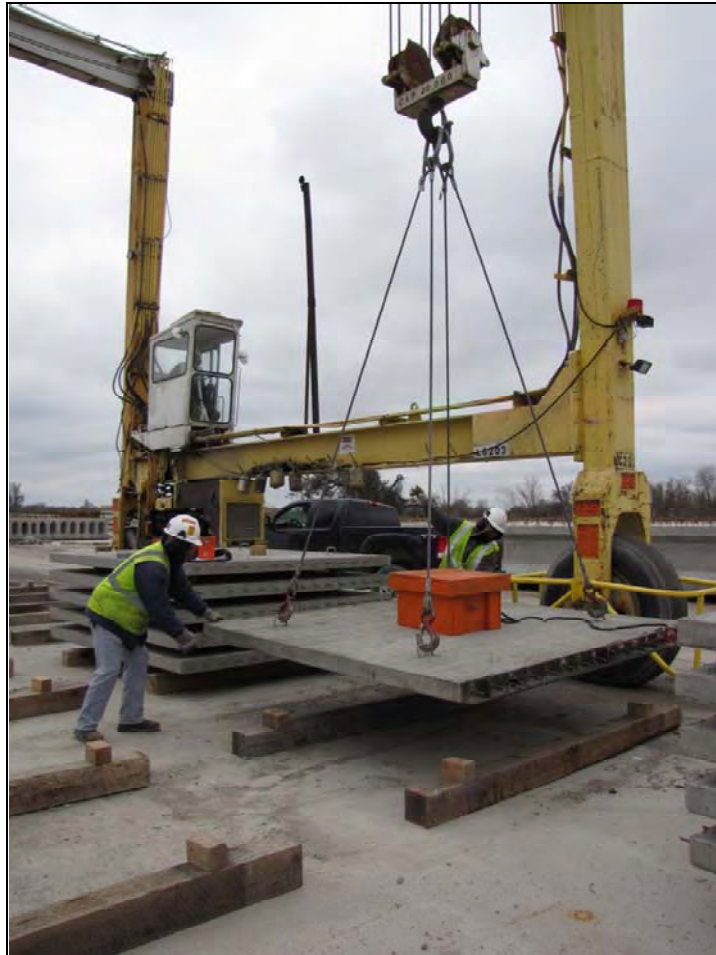
Figure 6.12 Stacked panels being placed in the storage area at Plant B
