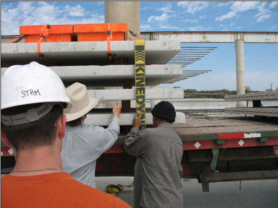
Figure 4.18 Side view showing relative alignment of straps and dunnage
