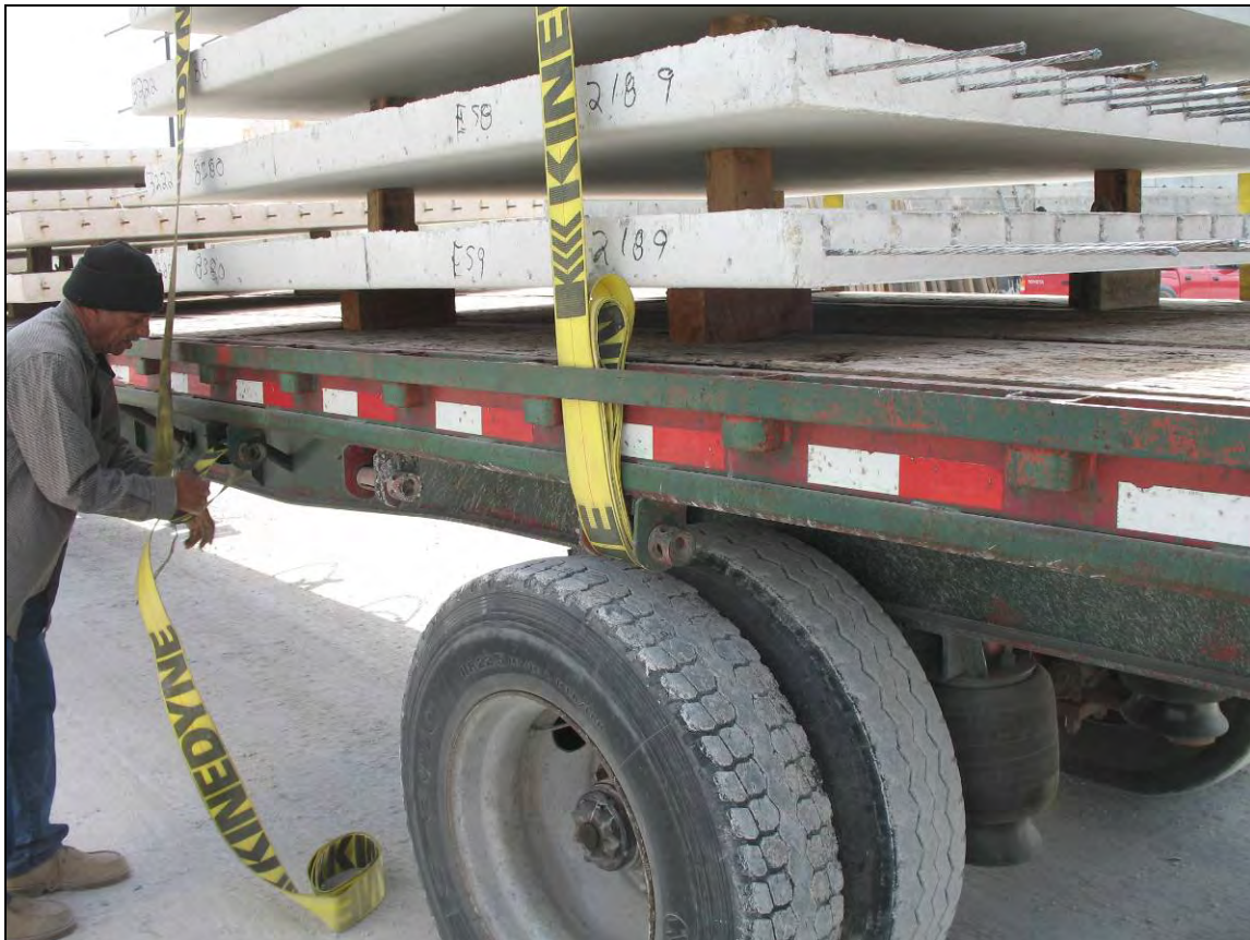
Figure 4.16 Panels strapped to flatbed truck
