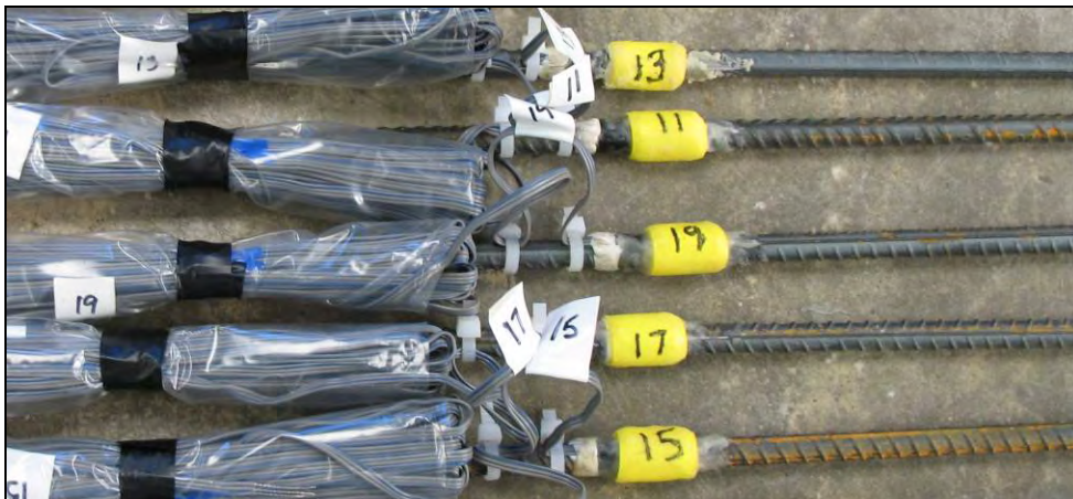
Figure 4.9 Set of gages completely installed on additional bars
